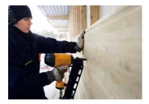
**Simple installation** A glulam panel is installed in exactly the same way as an ordinary panel, with nails or screws. Installation can be done even more efficiently by using panels which are end-tongued and grooved.
